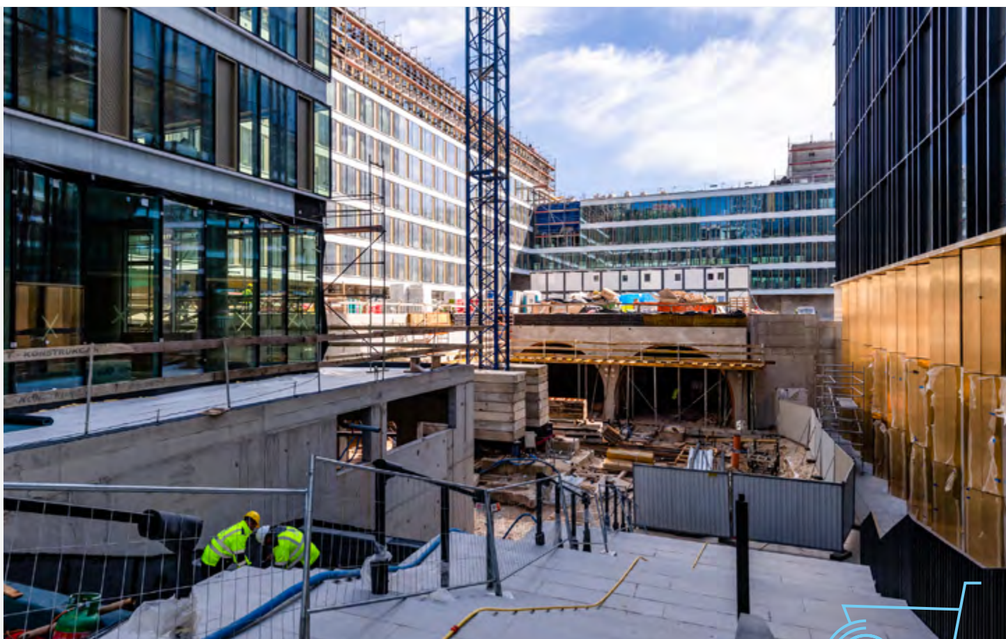
Construction works on the Malthouse Offices in the Warsaw Brewery complex
