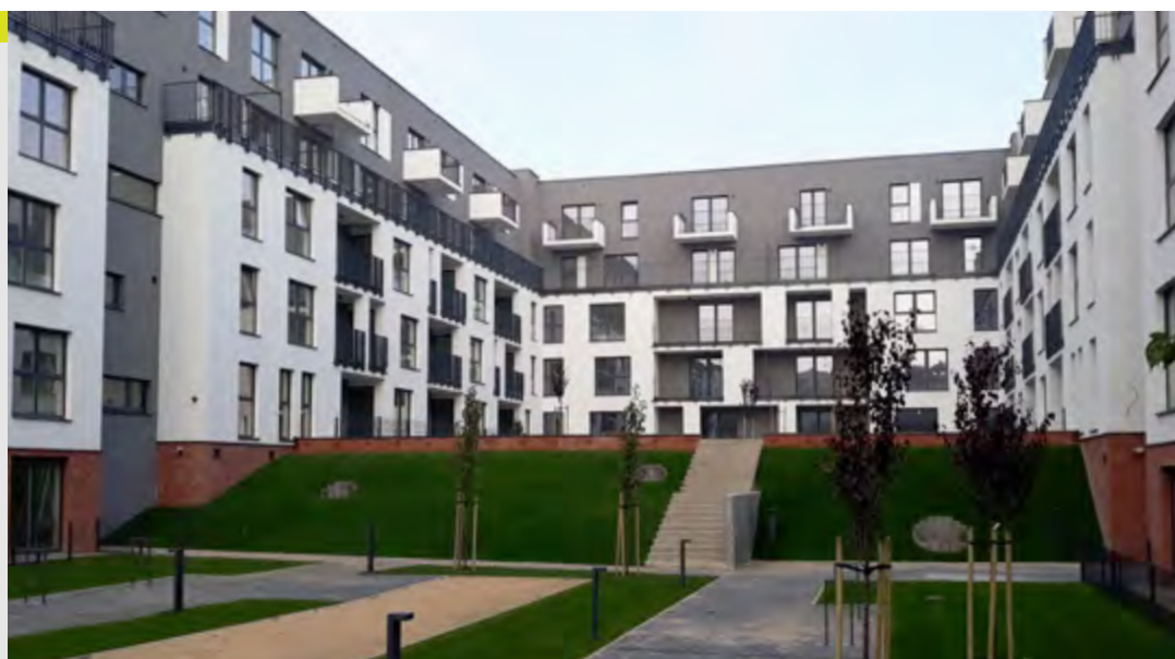
Recently handed over project in Łódź
